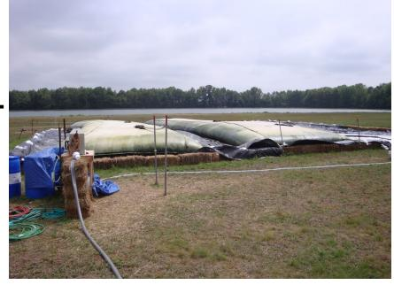
A Port-A-Poly polymer makedown system is set up near the bags. **Drainage netting** between the sheeting and bag provides additional drainage. At the back of the bag lay down area a sump collects the clear effluent that drains from the bags and it is pumped back to the lagoon with a gasoline pump.
