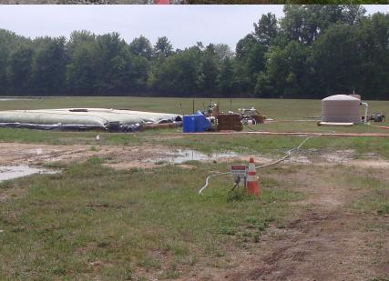
Three 45' circumference X 100' long dewatering bags are staged to accept the sludge. Room for an additional 3 bags is prepared in case they are needed. Polyethelyne sheeting is laid out under the bags.
