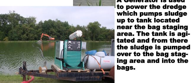
Dredging was done by using a stainless steel cable stretched across the lagoon. One end of the cable is fixed to the hydraulic hoe located on the far bank, the other hooked to the trailer that held the generator that provided power to the dredge. After each pass the hoe and trailer were moved about 4 feet to make ready for the next pass. Only one pass would be made across the lagoon. The travel speed is adjusted to reduce the sludge blanket to the desired amount.
