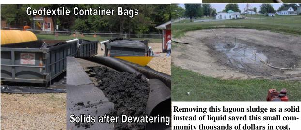
In this case the bag is set on the bank next to the lagoon. The sludge is pumped over and through a Blue River Technologies sludge flocculator where the chemical solution is mixed with the sludge flow. This causes the solids in the slurry to agglomerate and clear water to separate from the solids. In any geotextile process this is an essential step. Without good chemical mixing and addition the bag will blind over and the process will not be successful.
