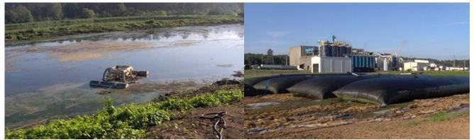
This food processing plant lagoon was pumped with a floating submersible pump pulled around to different spots with ropes. By moving the pump around most of the sludge was pumped over to the bags. Plastic Liner was used to divert the effluent that flowed from the bags back into the lagoon.
