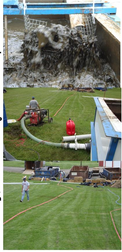
Each roll off is set on plastic and a containment area with straw bales collects the effluent that flows from the bag. It is directed to a sump and pumped back.
