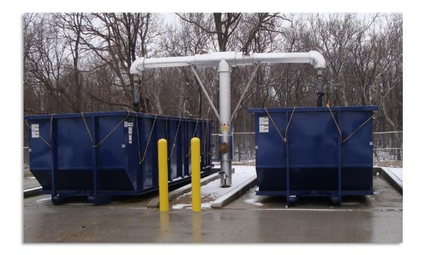
This type of system is used for plants that need a system always ready to pump without having to set up a flocculator and lay out hoses. The sludge is pumped thru the flocculator and out to the dewatering pad underground. Then it flows up through a stand pipe and over and into whichever roll off is in use at that time.
