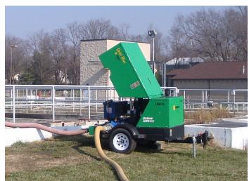
A Gorman Rupp pump is rented to pump the sludge from the rectangular holding tanks about 150 feet over to the drying bed area. The two large circular tanks also have a rental pump that is used to pump their contents over to the rectangular tanks as they are pumped down.
