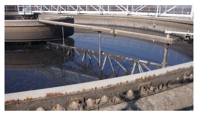
This tank has only a couple feet of sludge left in the bottom. All the sludge will be pumped into the geotextile bags. The tanks can be pressure washed and cleaned. The removal of over 1 million gallons of sludge will greatly improve the operation of this waste water plant and the operation was carried out in the most economical manner possible.
