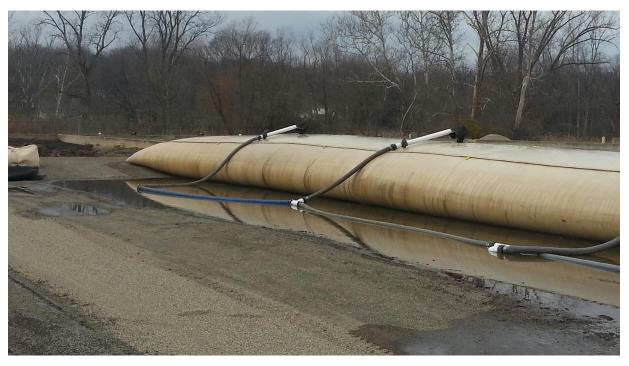
At this point in the process approx 400,000 gallons has been pumped into this bag. The sludge ranges from 1% solids to 1 1/2%. This bag can be pumped to a height of 6 feet. Then the pumping will be shifted to the other bag and this bag allowed to dewater a couple days before being pumped again. A second bag is to be laid next to this one now.
