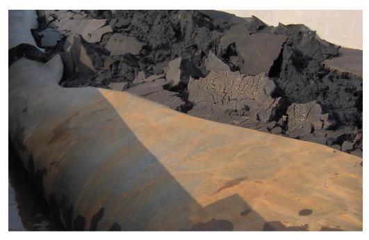
After the sludge pumping operation is completed, the bags will be left on the beds to dewater. They can be left on the bags as long as the beds are not needed. They can be opened and the sludge disposed of at the local landfill from as little as two weeks after the last pumping.
