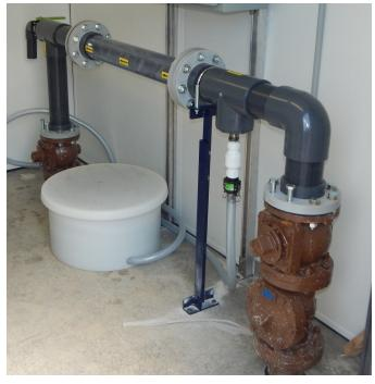
The hard piped flocculator assembly can be set up with a plug valve, and in some cases a flow meter will be installed to allow the operator to monitor flow rates and total flow thru the system. This allows very accurate record keeping of total gallons wasted per day thru the system.
