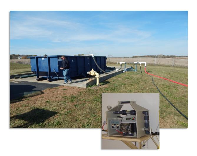
In this installation, a submersible pump is dropped down into the digester. This plant only needs to dewater 3-4 times per year.
